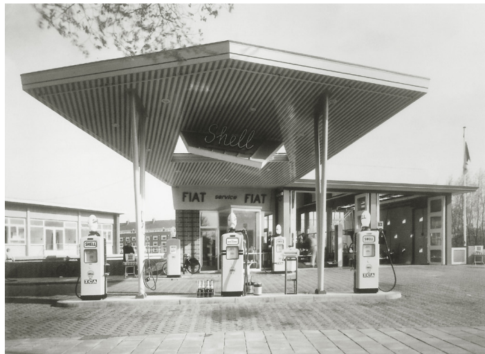
13. Shell service station [1954] with the original awning (which is replaced in the 70s.)
