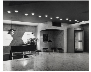
47. Interior of the Amro bank branch in the Waterlooplein project, with refined white marble and hexagonal shaped windows in the elevation, which are demolished.
