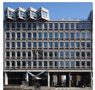
Metropolitan building shows prominent triangular roof structures and expressive awning
