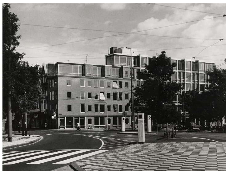
The elevation facing the Frederiksplein in the late 1960s, with some opened pivot windows.
