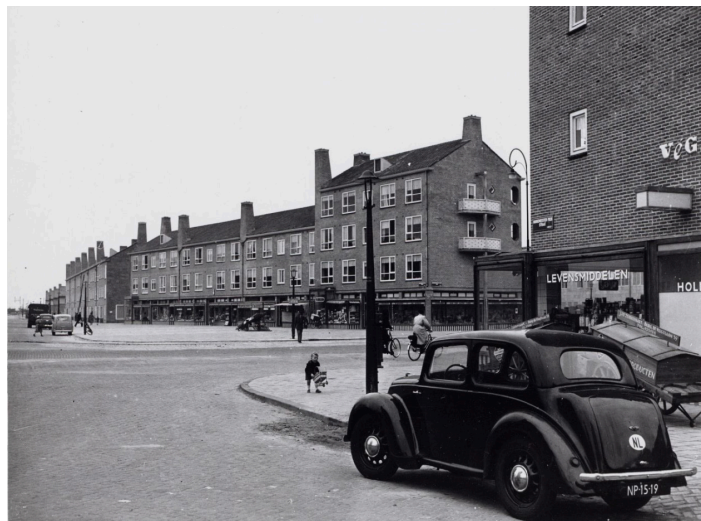
10. Post-war housing project with apartments and shops on ground level on Burgemeester Fockstraat in Amsterdam New West [1957].
