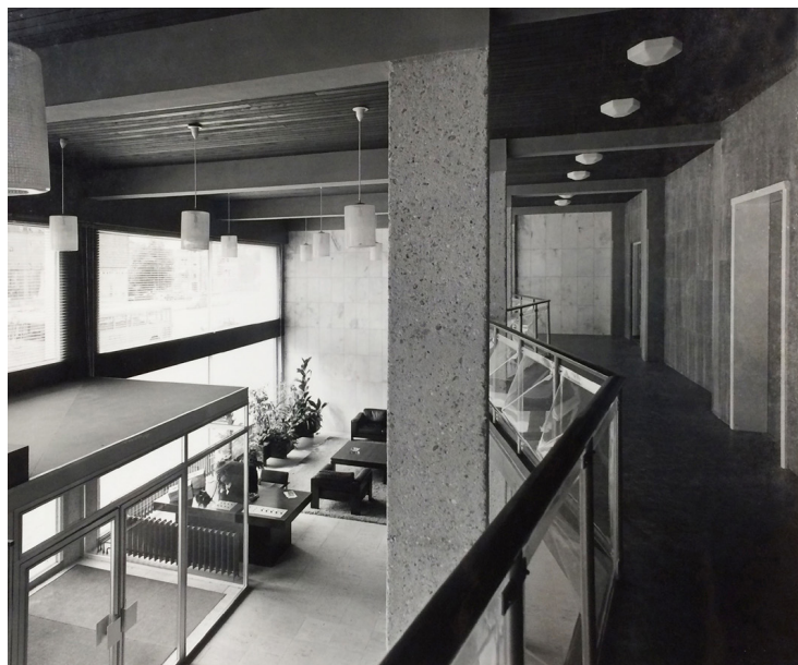
Entrance hall of De Metropool in its original state [1969].
