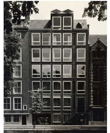
41. Office building at Keizersgracht 277 [1968].
